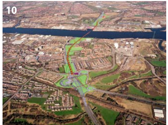
New Tyne Tunnels in Newcastle, UK
