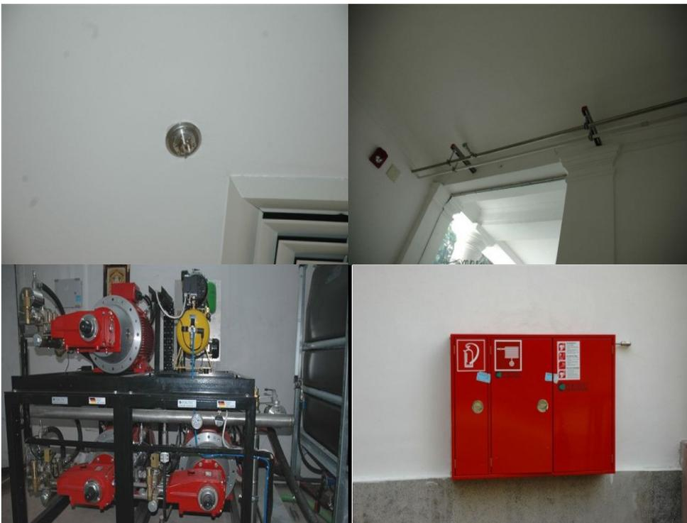
*Pre-action pump system with side wall nozzles and some parts of ceiling void have been protected. Also hose reel cabinet with FOGGUN 2 has been decided to place outside at strategically defined location.*
