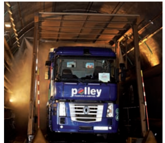
The 870 m long SAFE station has almost 900 mist nozzles spaced 2 m apart on each side of the train.
